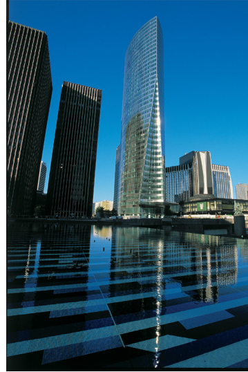
EDF TOWER - Paris, France 616,772 square feet
