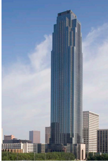
WILLIAMS TOWER - Houston TX 1,476,973 square feet
