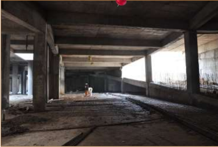
Reinforcement work, Drainage work & PCC work for Trimix
