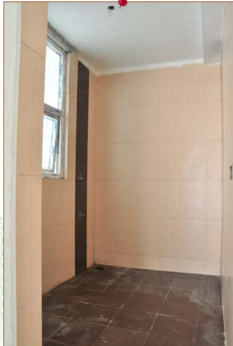
Ceramic tiles in wall & floor & UPVC window in Toilets
