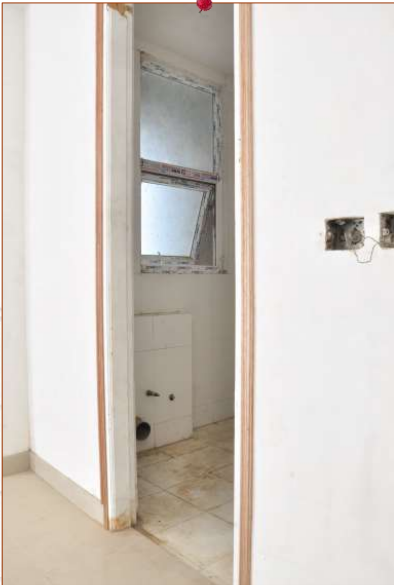
Wall & floor tiles ,wooden beading, UPVC Window in Toilets
