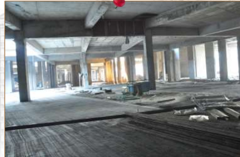
Trimix flooring work in basement area
