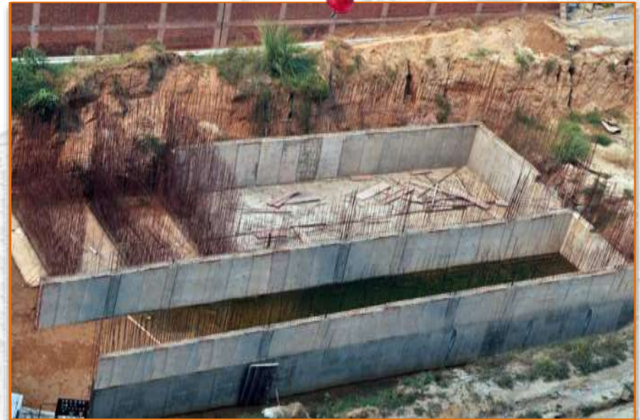
Construction in progress for S.T.P.
