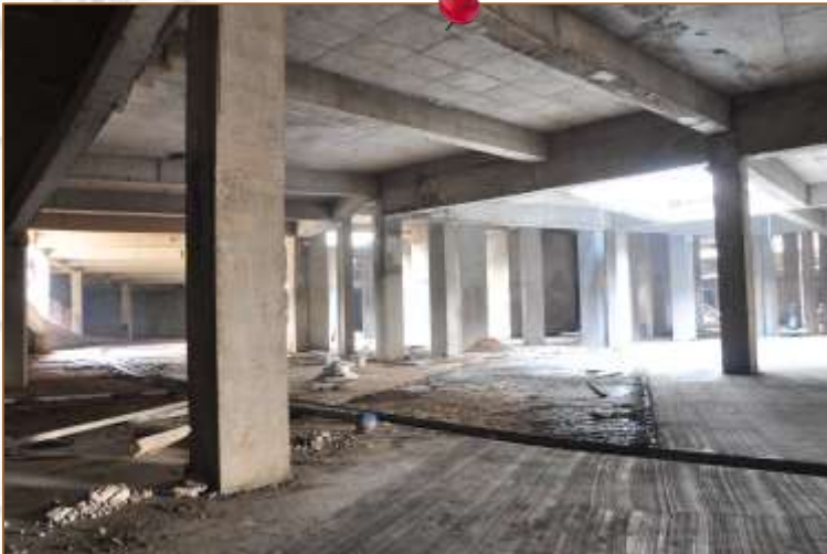
Trimix flooring work in basement area
