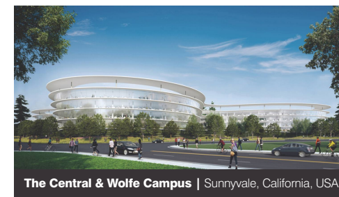
The Central & Wolfe Campus | Sunnyvale, California, USA
